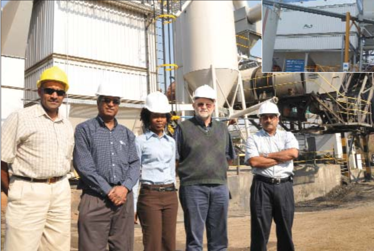
Above: The new baghouse at Much Asphalt Port Elizabeth, showing the dust extraction duct prior to painting.
