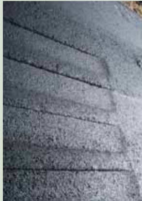
The trial section incorporating 55% recycled material.
