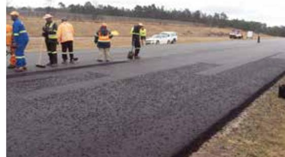
Semi-gap mix with overlay of pre-coated chips.
