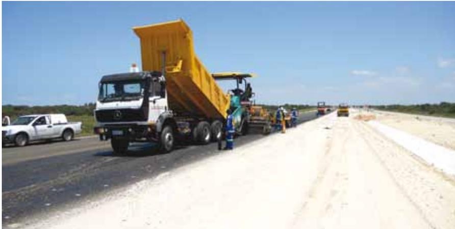
Paving of semi-gap mix on the N2 Colchester project in January 2012.
