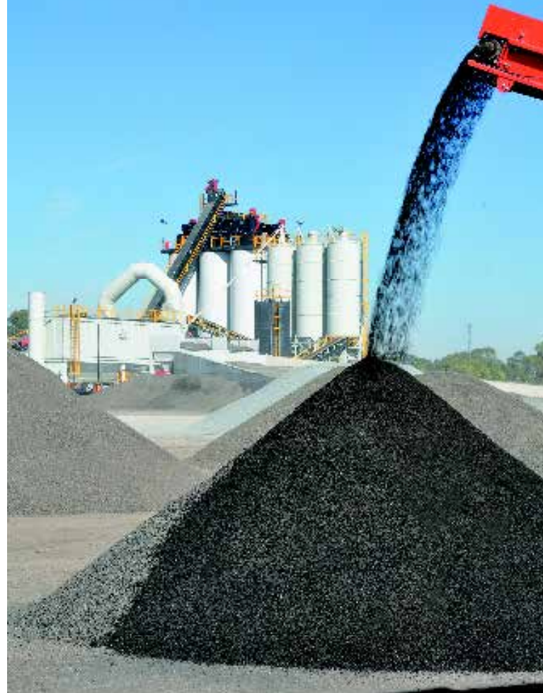
Fine RA feeding from screening plant
